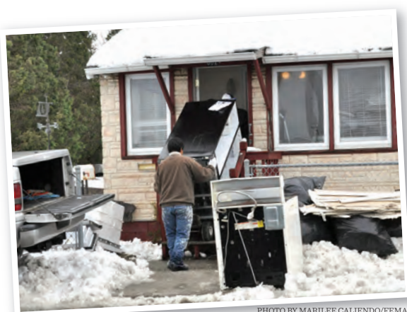
A storm-damaged home in Milford
